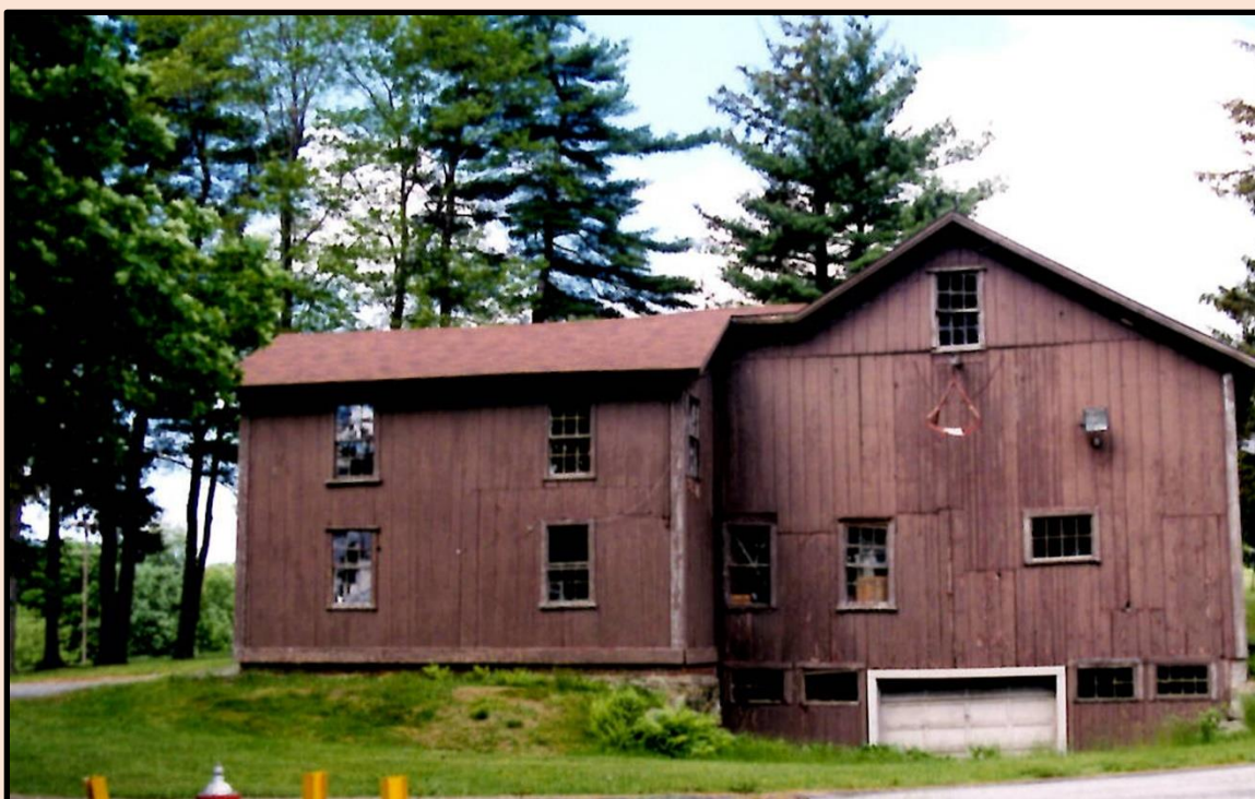
Red Barn at Hillside
